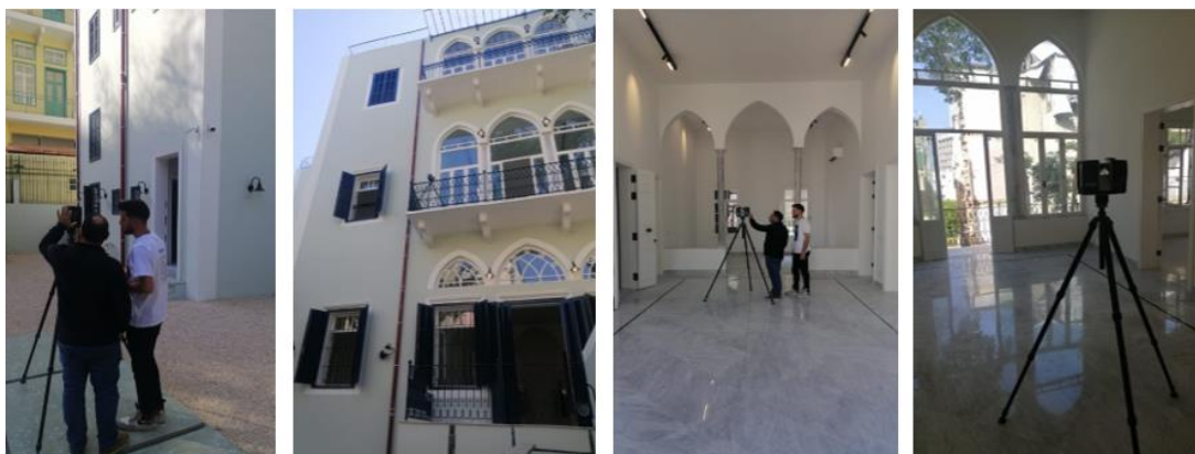
Fig.16 a, b, c & d: TLS survey process for HBIM of the block Rmeil 695 Source: Jawad Chamoun, Ralph Khoury.
