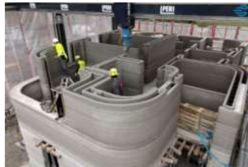
Figs.43 & 44: The 3D Printing process
