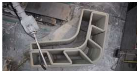
Fig.24: 3D printing on site work
