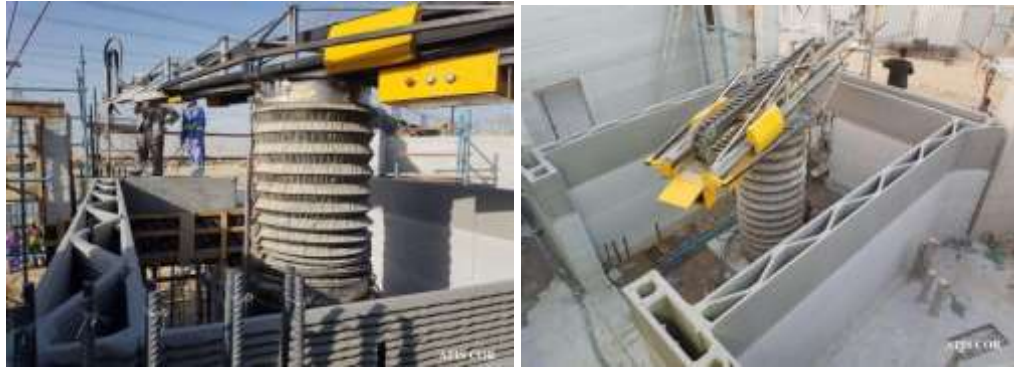
Figs.37 &amp; 38: 3D Printer used from Apis Core
