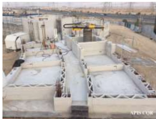
Figs.35 & 36: Dubai municipality 3D Printing process
