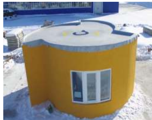
Fig. 20: 3D printed livable house in Russia Source: https://www.boredpanda.com/
