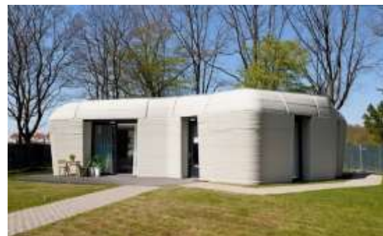
Fig.23: 3D printed livable house exterior view.
