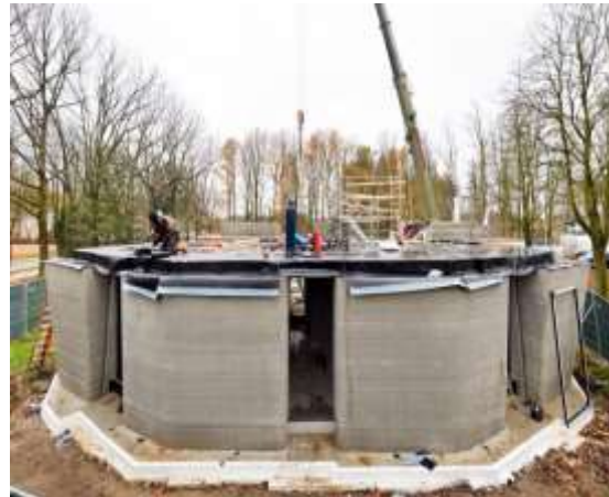
Fig.25: 3D printing process
