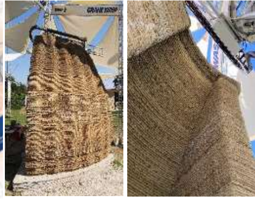
Figs.28 & 29: 3D printing process of TECLA
