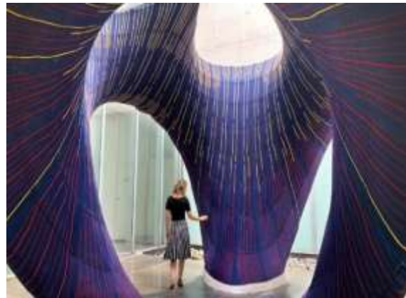
Fig.15: KnitCandela - A flexibly formed, thin concrete shell at MUAC, Mexico City Source: RocketshipWP, 2018
