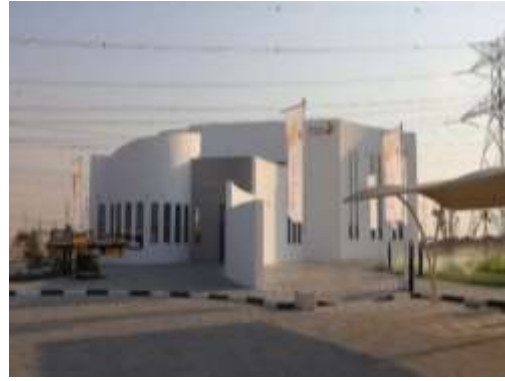
Fig.34: Dubai municipality external view
