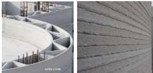
Figs.39 &amp; 40: Steel columns inside layering by human intervention
