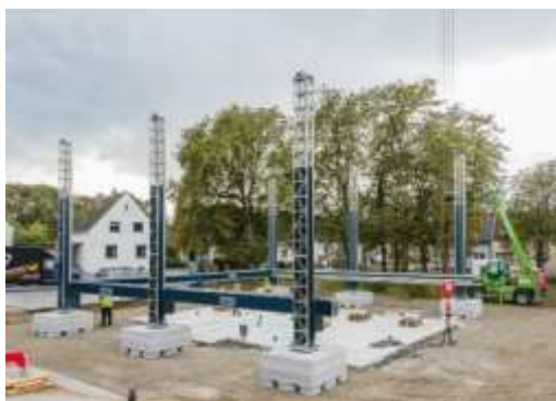
Fig.45: The 3D printing of foundations
