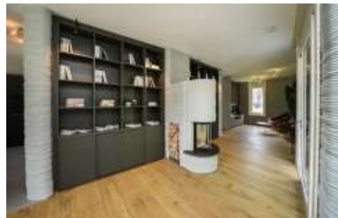
Fig.47: The interior showing the chimney created also layer by layer.
