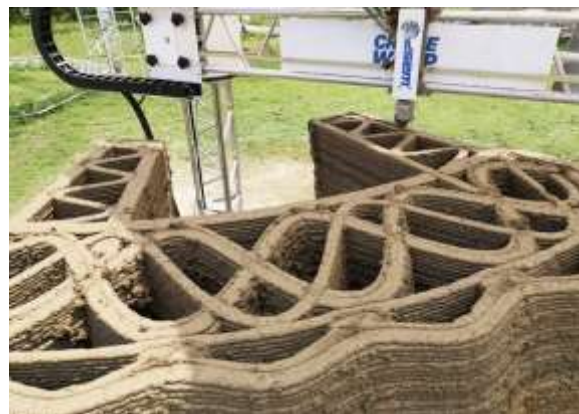
Figs.30 & 31: Undulating curved layers provide structural stability.
