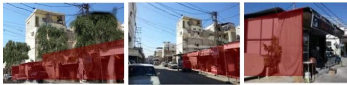
Fig.27: Pictures shows the unusable stores in the Sekkeh Street.
