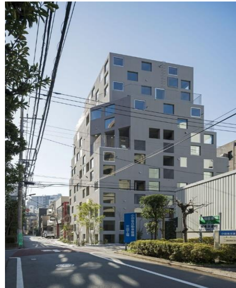
Fig.29: residential building concept and plans of “Hatsuse Mita Apartments” Source: “Inatsugu Taisuke, 2020”.
