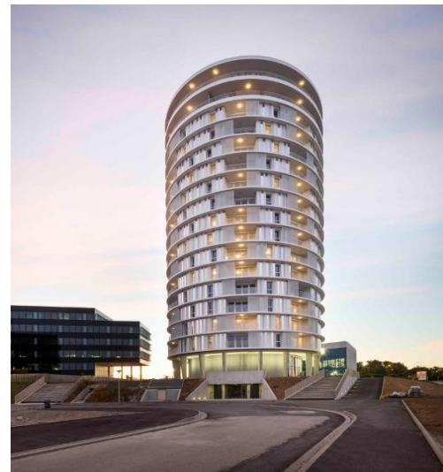
Fig.20: exterior photograph of “Tour Lumiere”
