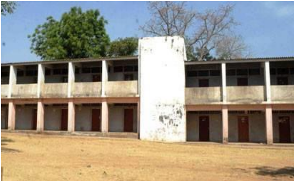
Fig.4: Showing a view to the hostel entrances with doors and windows in place for ATBU Source: Author, 2021
