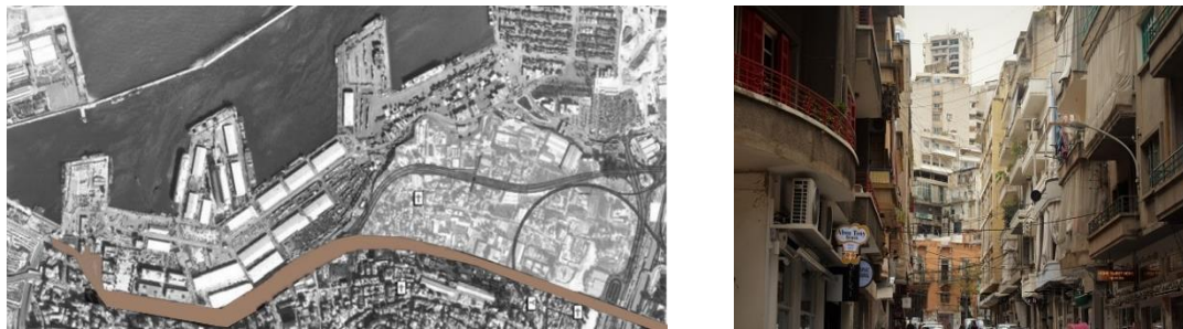
Fig.19: (a) On the left, The Charles Helo Highway separating Mdwwar neighborhoods (Source: Google earth), (b) On the right, Crowded neighborhood in Medawwar
