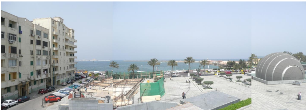
Figure 5: Panoramic view of the new building under construction.
