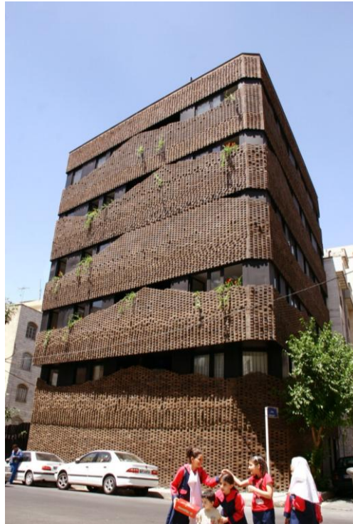
Fig. 7 North-east view Source: Author Nov 2013
