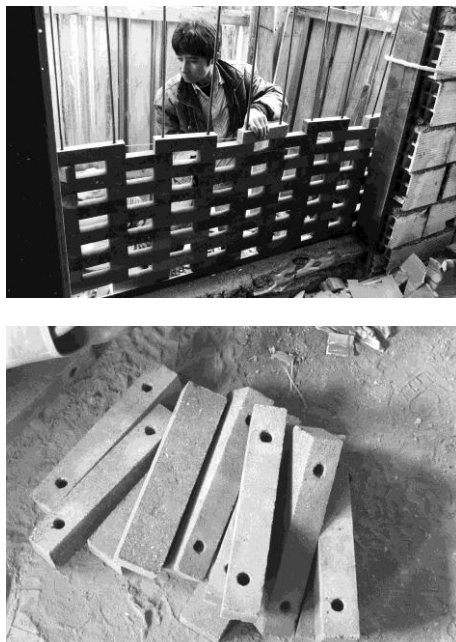
Fig. 5 Preparing bricks for brickwork Source: Author March 2013
