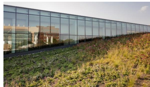
Fig.24: Green Roof and Outdoor Terrace in Charles Library at Temple University (“The library of the future is here,” 2019) (“New library receives state support for massive green roof,” 2016)
