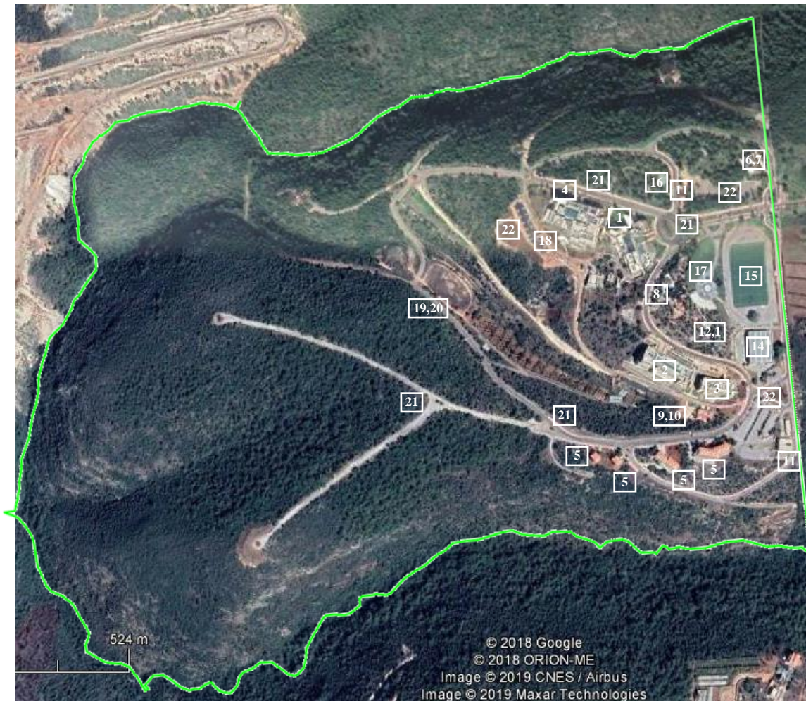
Figure 9: The Debbieh Campus (Case A) (numbers refer to the site contents, see Table 6) (Google, 2018) (Source: Author)
