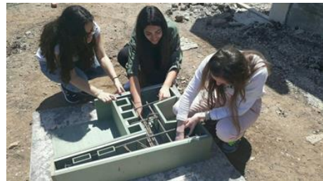
Figure 4: Concrete form preparations Source: by authors.
