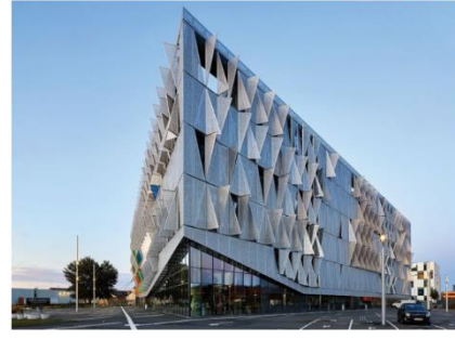
Fig. 8 shows the ADU building when its panels are open (Source: Stephen, 2015)
