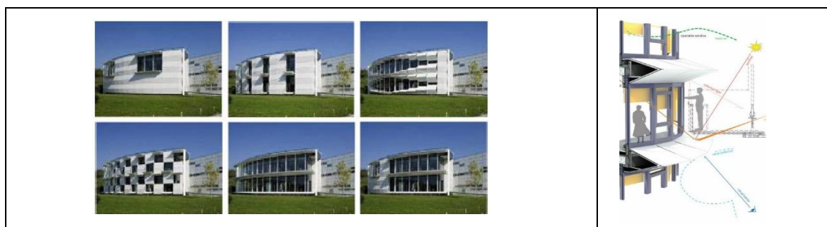
Fig. 6 Aluminum panels operation of Kiefer Technic Showroom (source: fouad, 2012)
